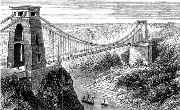
Clifton Suspension Bridge
